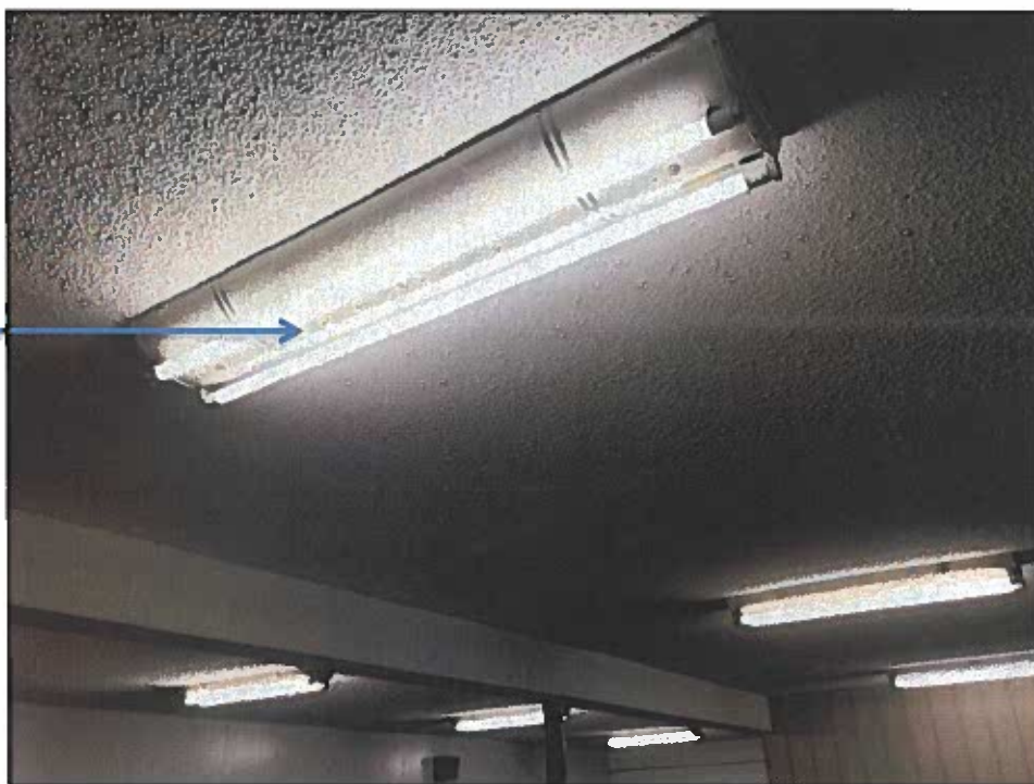
Photograph #5: Suspect PCB-containing light ballasts and mercury-containing bulbs/lamps – Throughout building
