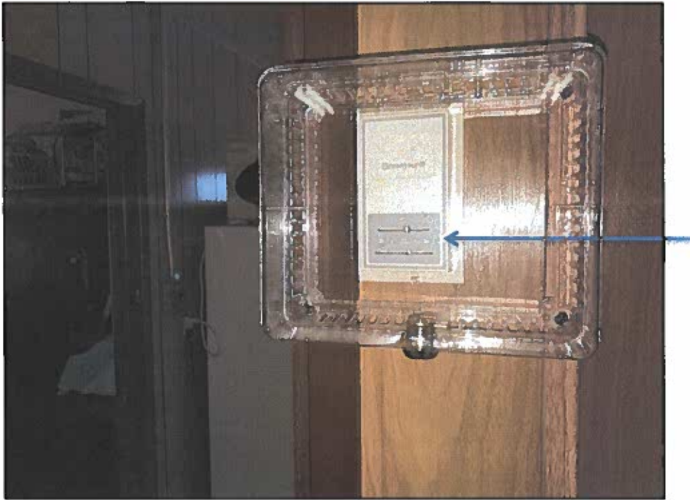
Photograph #9: Mercury-containing thermostats – Throughout building
