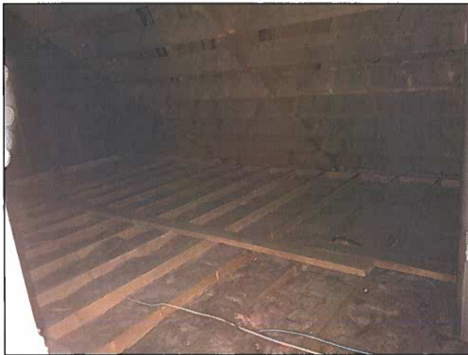
Photograph #10: Fibreglass batt insulation within main floor attic spaces
