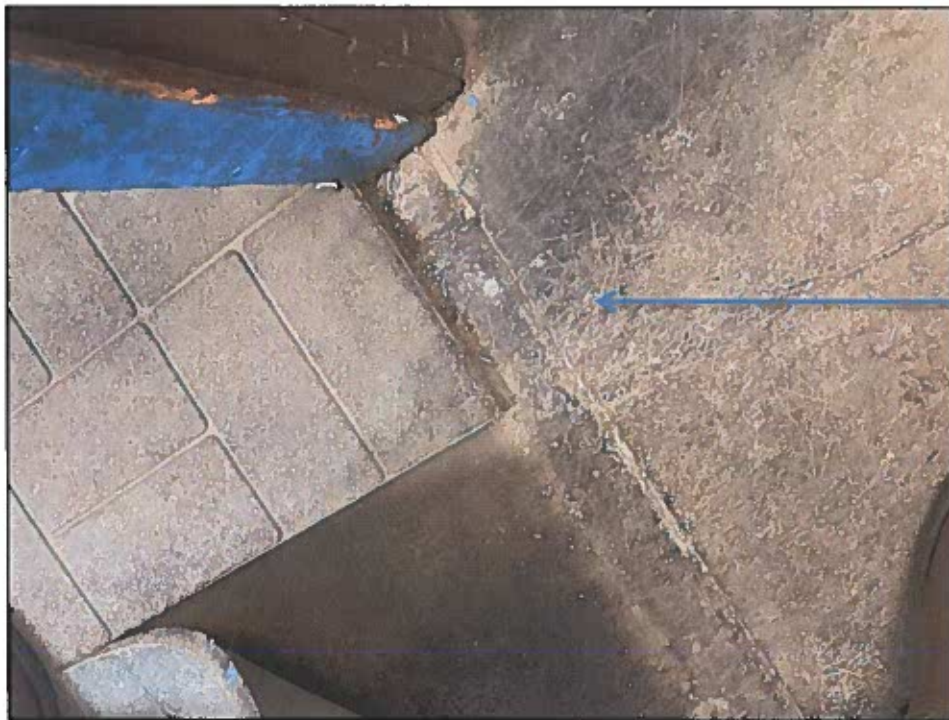
Photograph #2: Asbestos-containing 1'x4' black skate-safe flooring planks (under newer rubber flooring) – Throughout Main Floor lobby/dressing room areas
